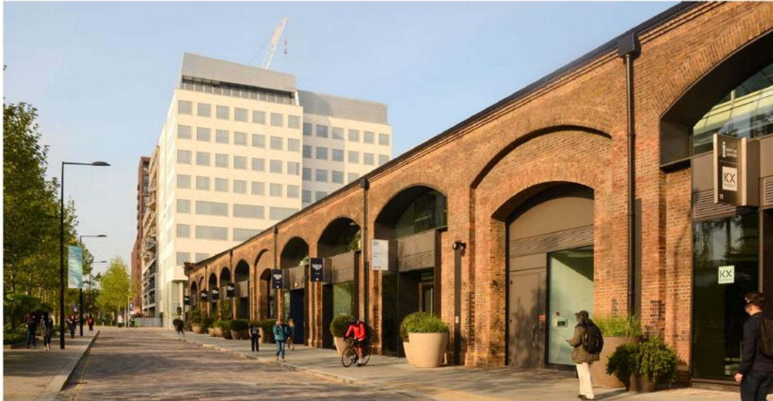
The Western Transit Shed
